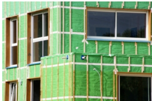
External solid-wall insulation
