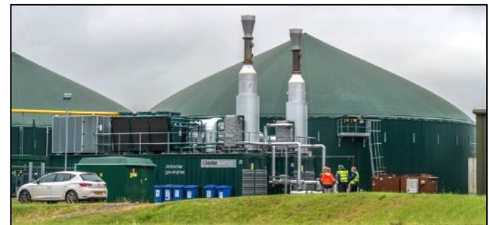
Agrivert food-waste digesters and 2.4 MW generators, Crowmarsh, Oxon
