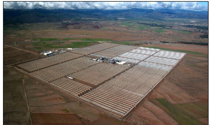
Andasol 150 MW concentrating solar power plant (parabolic troughs, molten salt) near Guadix, Spain
