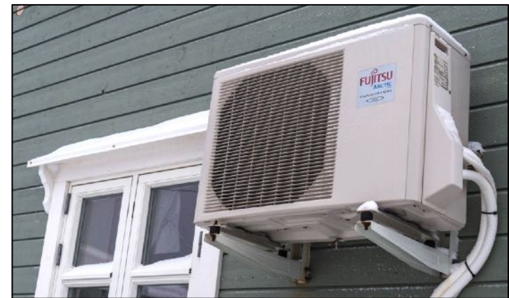
Air-source heat pump, Arctic Norway (70°N)
